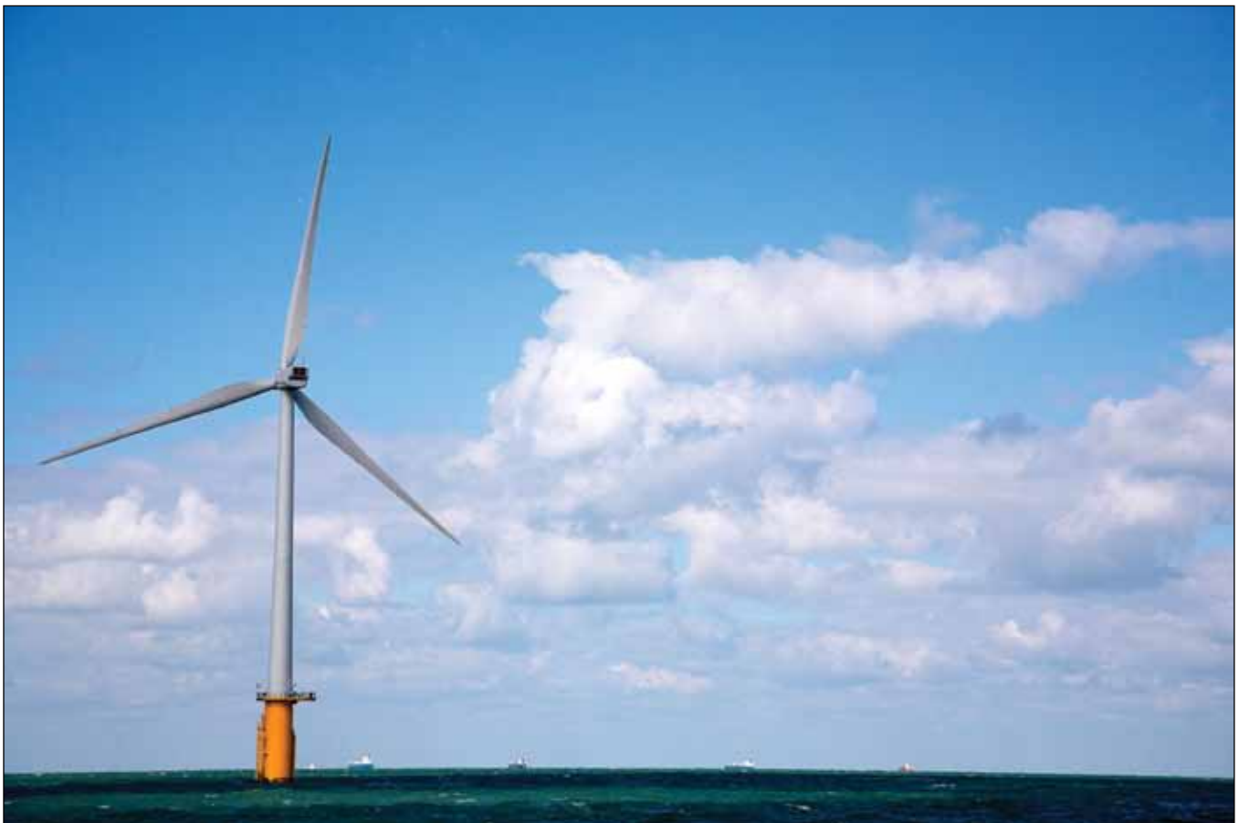
The Thanet project was completed in September 2010 and will boost offshore capacity by 30 percent (courtesy of Vattenfall).
