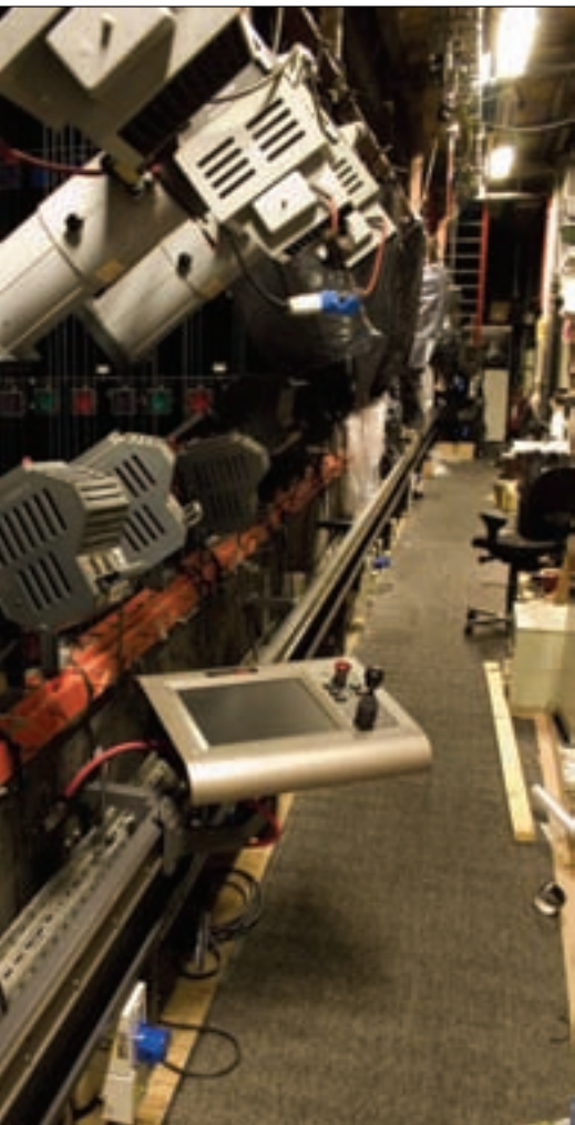
Visual Act's Touring Desk control panel is one of four portable control desks (courtesy of Sprint Electric).
