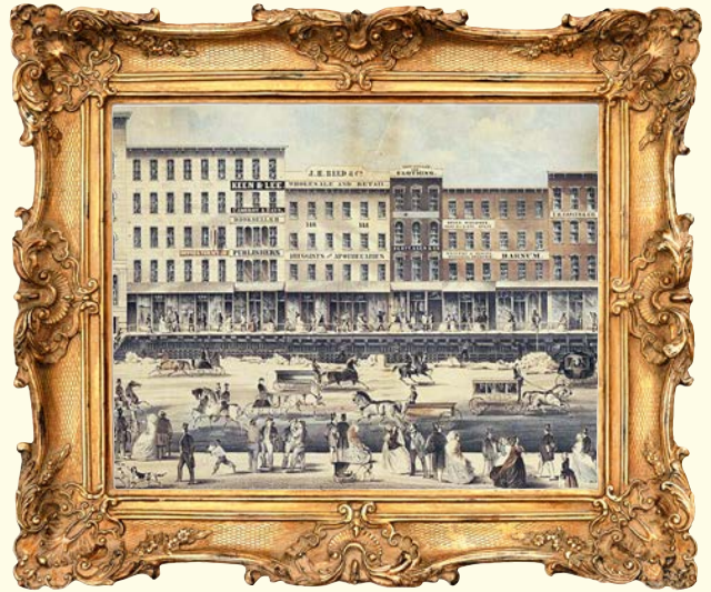
Raising a block of buildings on Lake Street (Photo Wikipedia).
