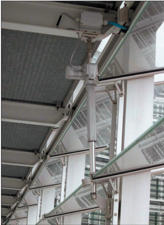
SKF actuators control positioning of window sun blinds.
