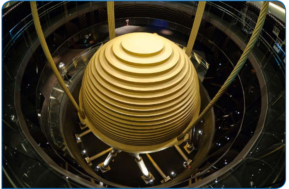
Tuned mass damper on display in Taipei 101. Photo by Armand du Plessis (CC BY 3.0)
