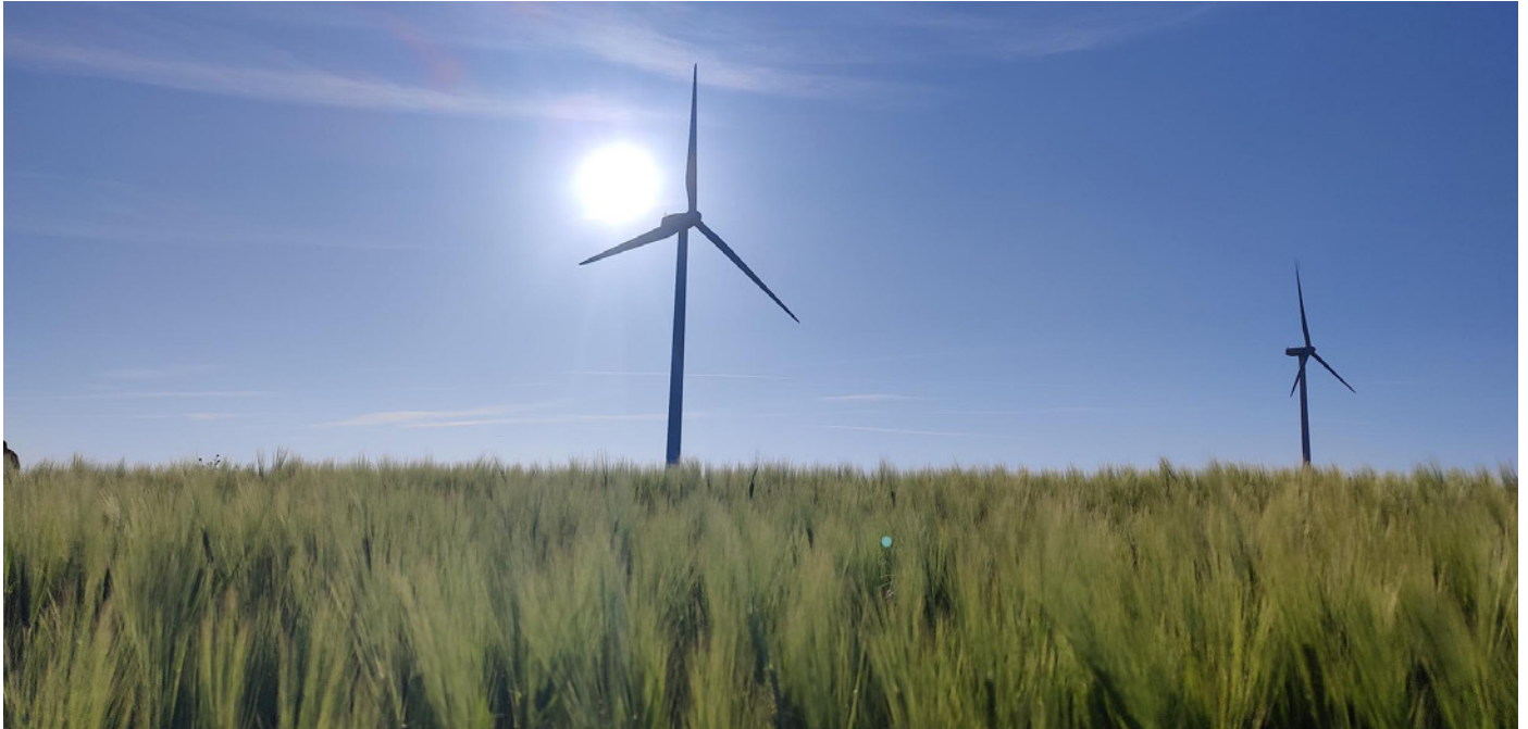
Condition monitoring systems can identify wind turbine issues before they worsen. All photos courtesy of ONYX InSight.
