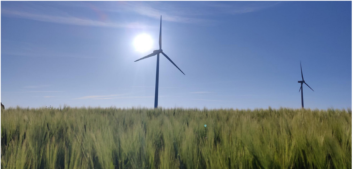
Condition monitoring systems can identify wind turbine issues before they worsen. All photos courtesy of ONYX InSight.
