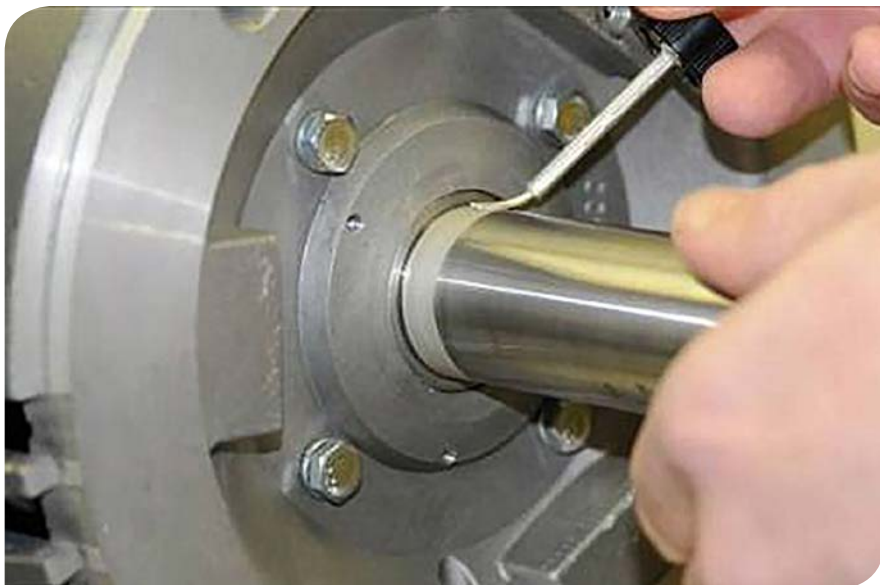
Figure 4 Prior to installation of a grounding ring, the motor shaft must be cleaned down to bare metal, free of any nonconductive material. Conductivity can be further enhanced by coating the part of the shaft that will contact the ring with colloidal silver.
