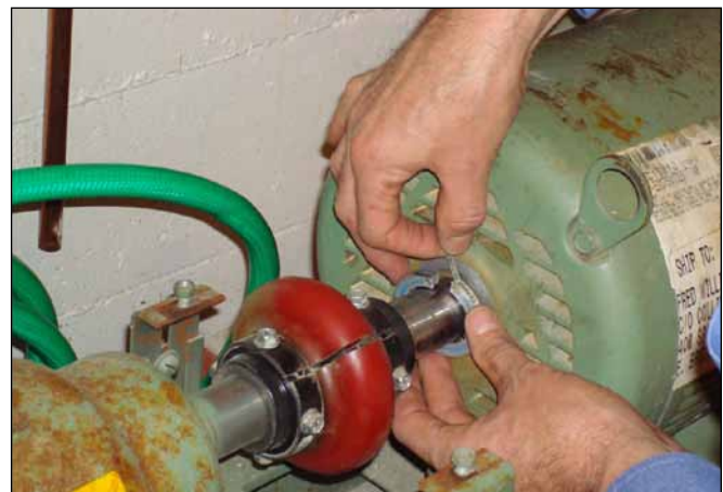
Figure 4—Ring is pushed back against bare metal of end-bracket, maximizing electrical contact via conductive epoxy. To ensure ring is correctly centered on shaft, metal spacers (included in the kit) are inserted into gaps between two halves of ring. Post adhesive cure, spacers are removed. Installation time: about 10 minutes.
