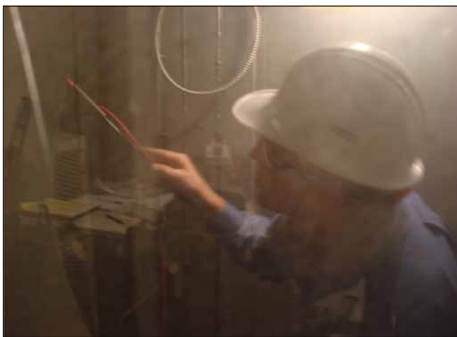
Figure 6—Unlike Motor #1, the Motor #2 shaft is difficult to reach, with only a couple of inches between the end-bell and a sheave exposed; the versatility of the splitting-ring Aegis SGR and ease of installation using conductive epoxy become even more apparent.
