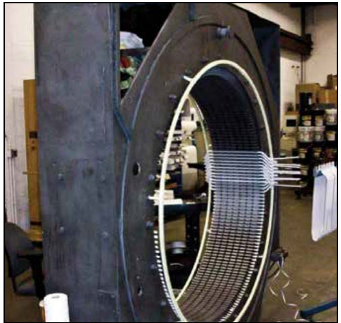
Figure 4 Five-hundred-horsepower motor undergoing new copper coil insertion (photo courtesy EECO).
