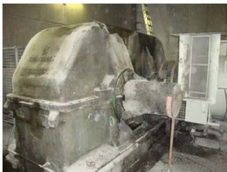
Figure 2 Two-stage reduction gearbox.
