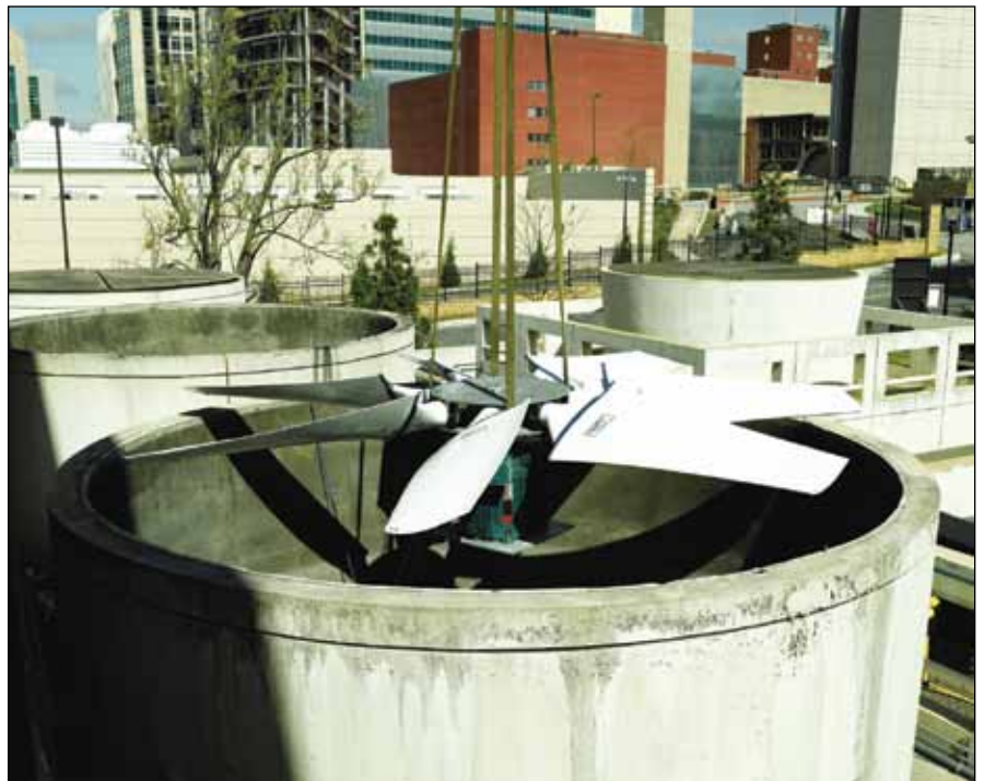
The Baldor Reliance RPM AC Cooling Tower Direct Drive Motor is designed exclusively for the cooling tower industry. This motor combines the technologies of the power-dense, laminated frame RPM AC motor with high performance, permanent magnet salient pole rotor designs (photos courtesy of Baldor).
