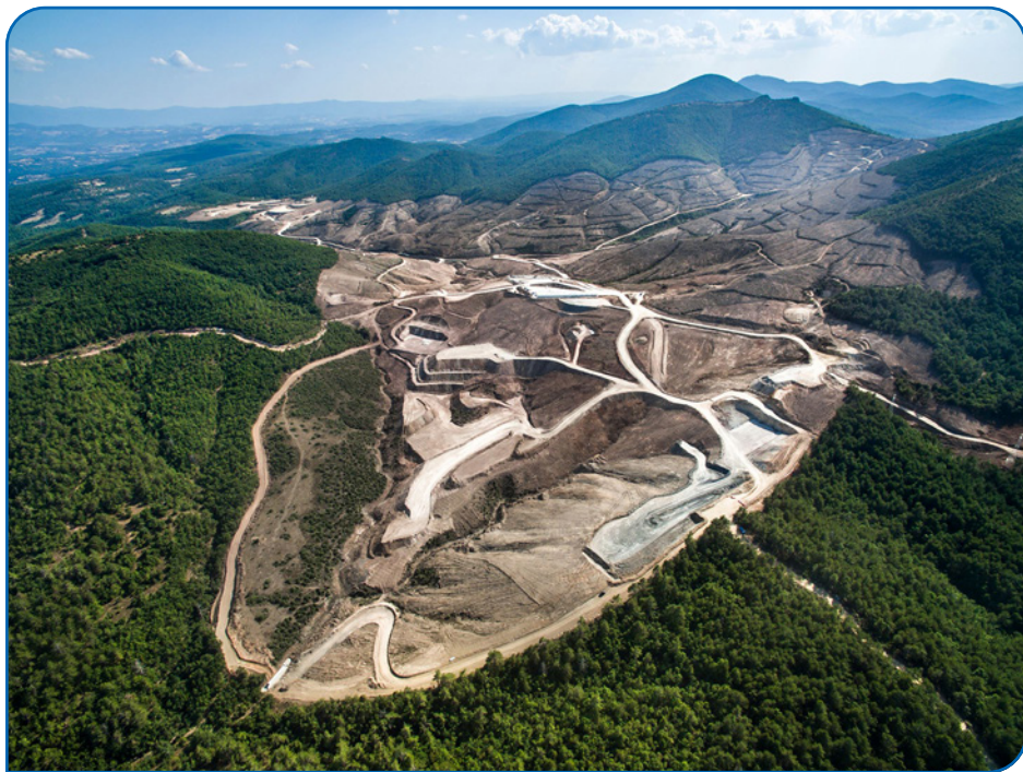
Mining site (Courtesy of Sulzer).
