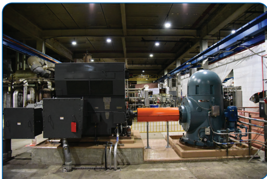
Philadelphia Gear drivetrain system includes new electric motor, right-angle pump drive, and control system.
